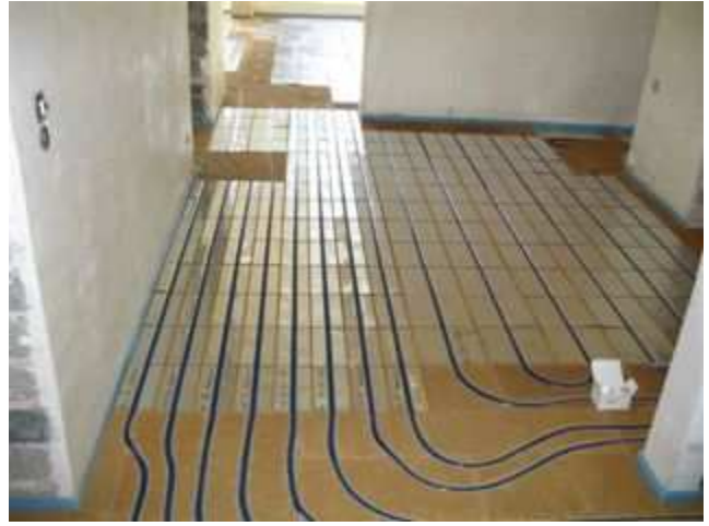
Area showing panels with 12.5 cm and 25 cm pipe centres
