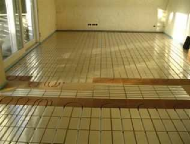
JUPITER panels in position ready for heating pipe
