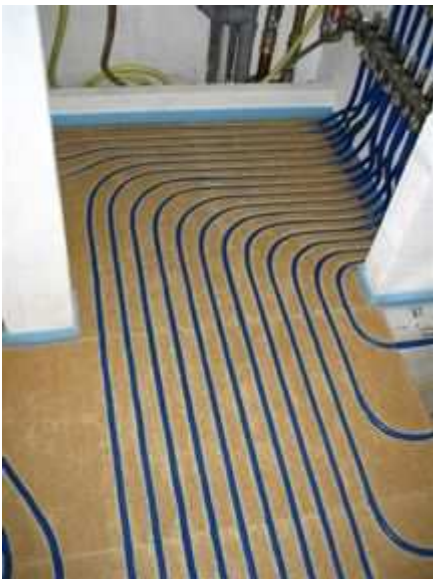
Hand routed channels for heating pipes leading from manifold
