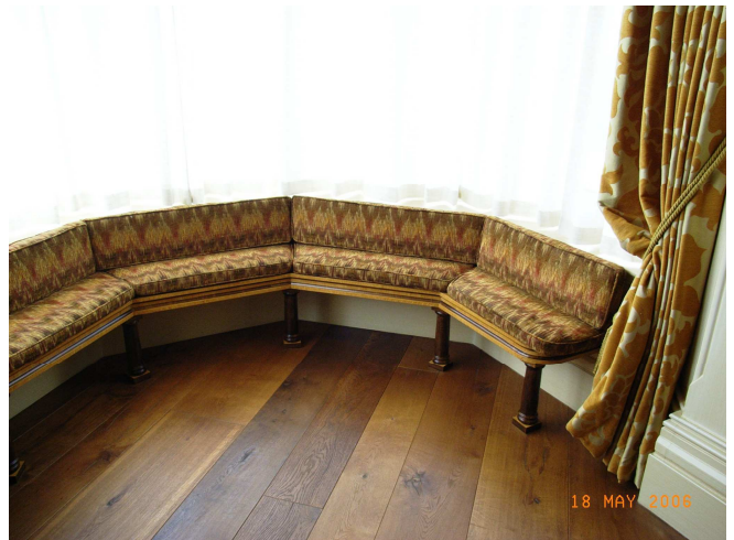
Schotten & Hansen timber floors installed directly over existing floor joists.
