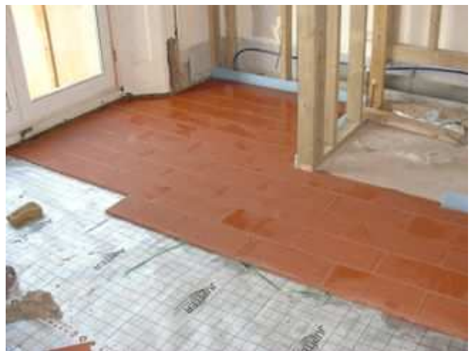
T&G Screed Replacement tiles laid directly on top of System panels (separating foil protects pipes from glue). Tiles act as load bearing surface for final stone floor.
