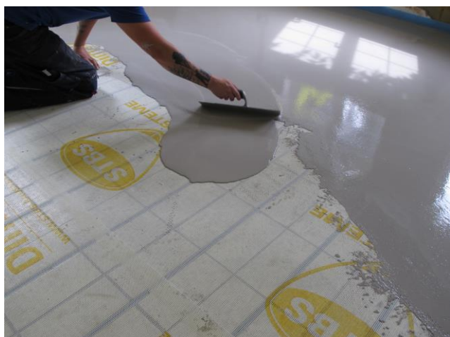
The MortaColl can be evenly distributed using either a smooth or notched trowel.
