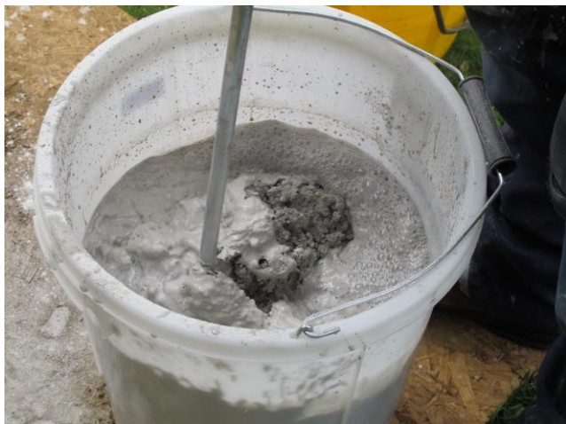
The thin screed supplied, MortaColl is mixed with water and reinforcing fibres.
