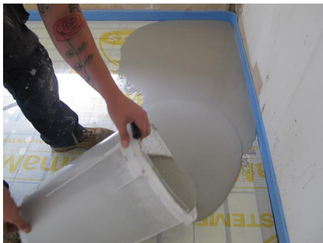
Once well mixed, the viscous mixture is gradually poured out over the DimaMat.
