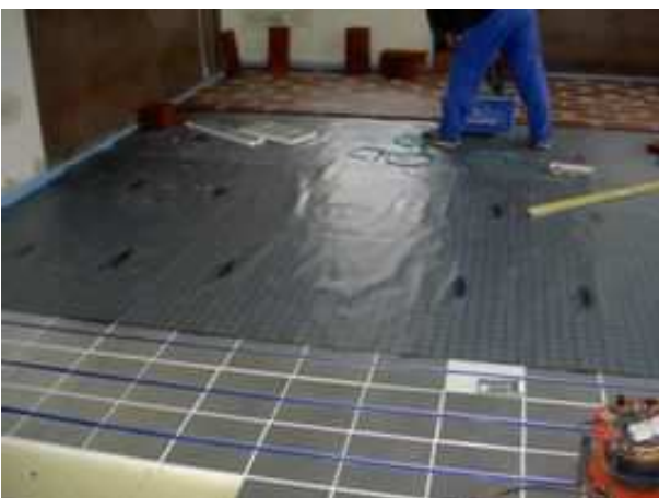
20mm Screed Replacement Tiles are glued together on a foil which prevents the tile glue coming in contact with the heating system.
