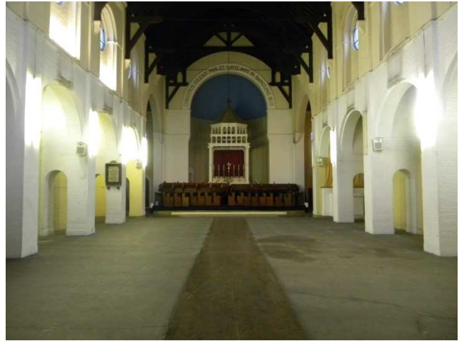
Fortunately the existing floor was flat and level enough to accept the JUPITER IDEAL system as soon as the pews were removed.
