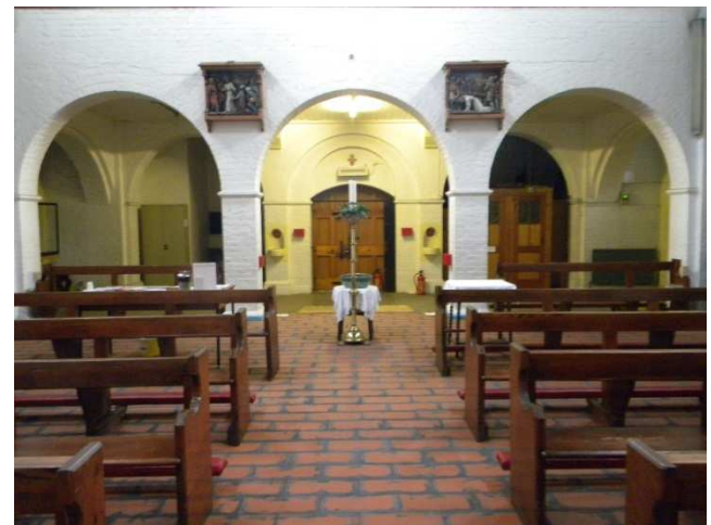
As a stop gap the Screed Replacement Tile substrate was used as a temporary surface before the final stone is installed.
