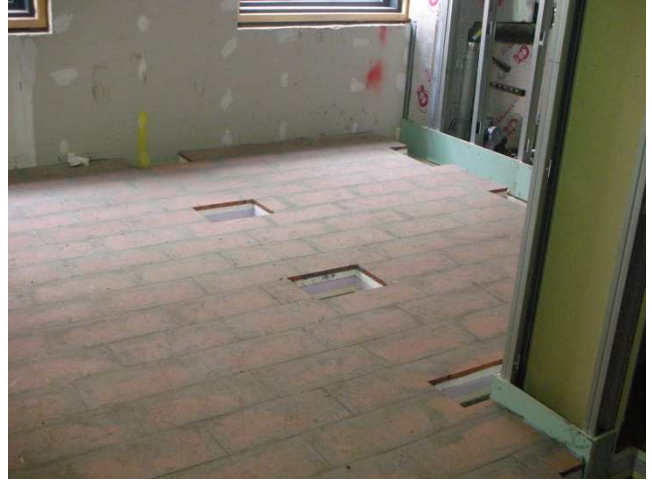
As part of the complete refurbishment of the Grosvenor House apartments, JUPITER were contracted to construct all bathroom floors complete with fall for wet room floors.
