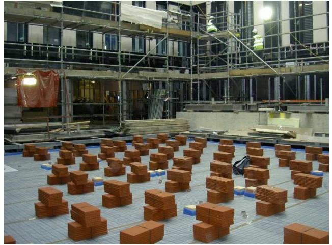
As part of the complete refurbishment of the Grosvenor House apartments, JUPITER were contracted to construct all bathroom floors complete with fall for wet room floors.
