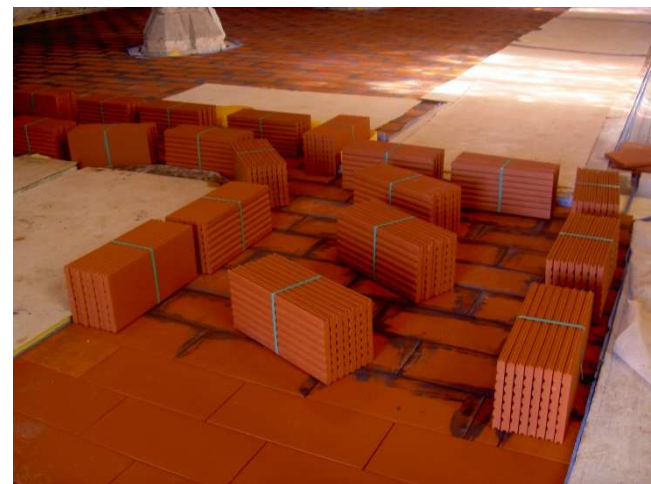
Screed Replacement Tile used as substrate for stone floor.
