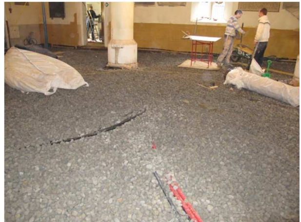
Haspor Foamed glass installed as main void filler. Depth approx. 300mm.
