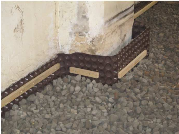
Edge detail showing tanking membrane holding limecrete border in place..
