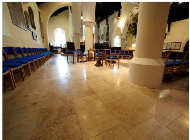
Installed stone floor. No intermediate expansion joints – total area 230m².
